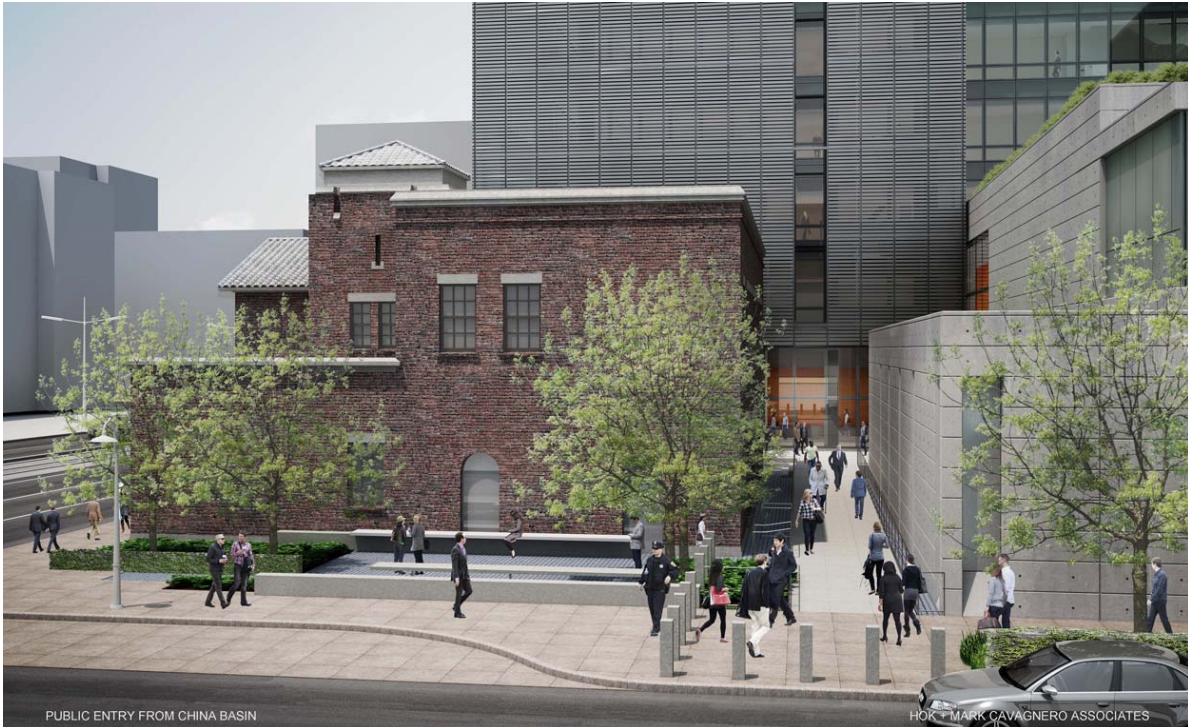
View of Fire Station along China Basin
